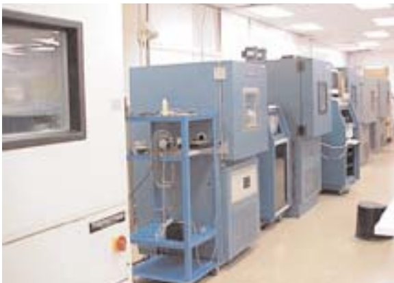
Riverside Reliability Test Facility
